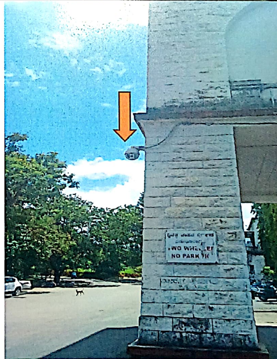
MAIN BUILDING CCTV SURVEILLANCE
